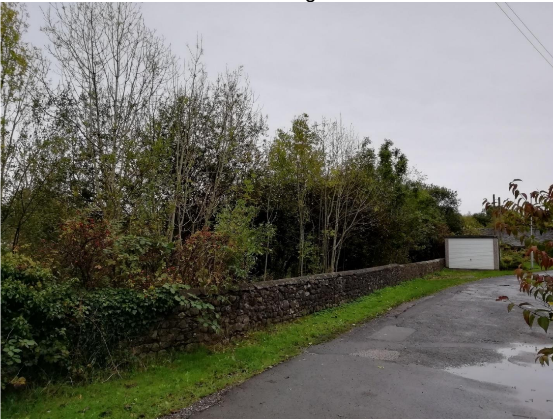
View of W1 from Carlisle Terrace looking westerly.
